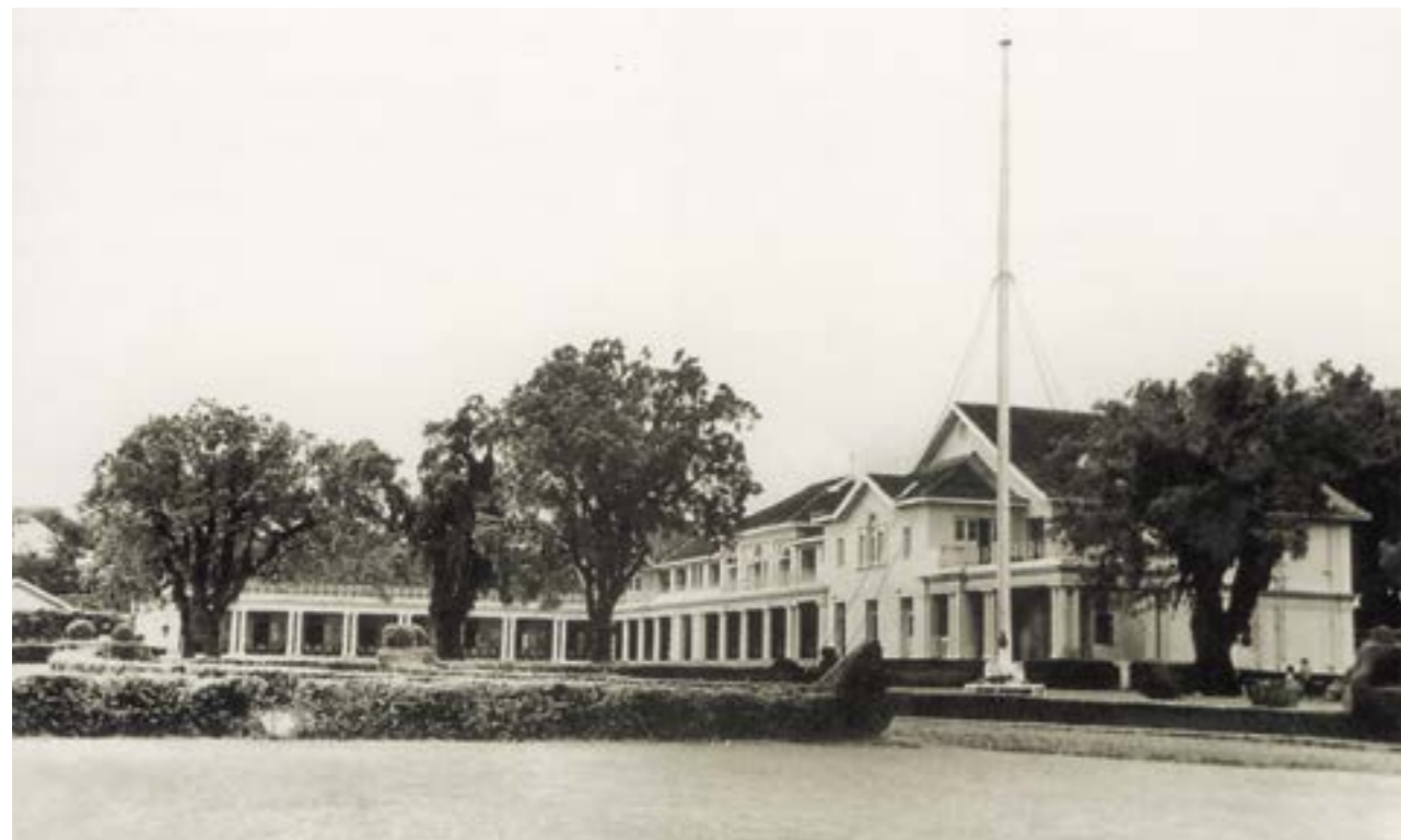
Turf club house for which the foundation was laid in 1918
